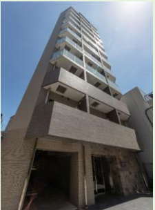
S-RESIDENCE Mita keidai mae Minato-ku, Tokyo 29 units
