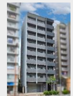
S-FORT Shin Osaka East Higashi Yodogawa-ku, Osaka-shi 25 units
