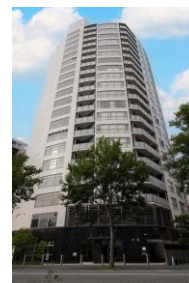
S-FORT Kego Tower A Rank ★★★★
